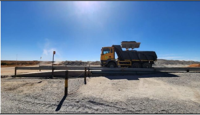
FORMALISED BUND AREA
